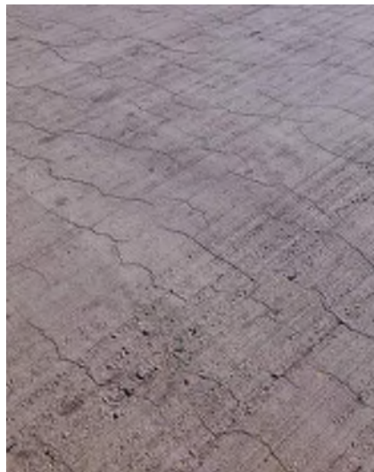
Figure 1.2 - Plastic shrinkage cracking in concrete.
